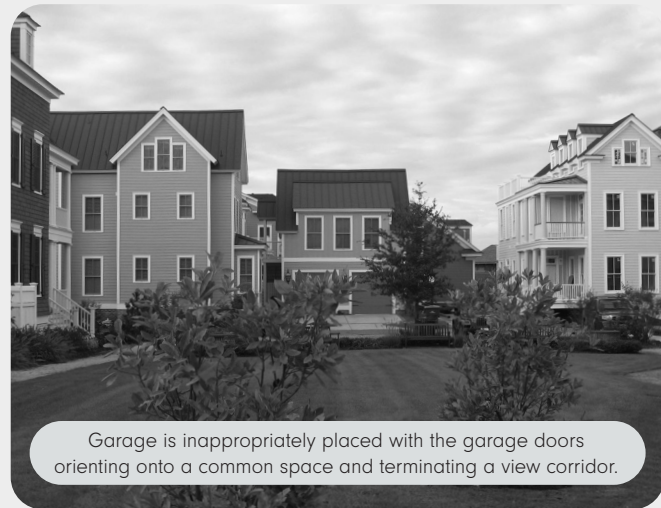
Inappropriate architectural character, massive irregular form and a lack of appropriate detailing fail to address the secondary street facade.
