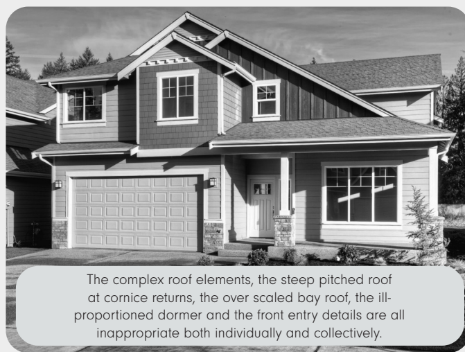
This example appears more like two homes joined by an over scaled entry element, lacks a sense of order, is overly complex, and is inappropriate.
